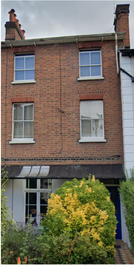
Front of no. 33 with 1 st and 2 nd floor timber windows
