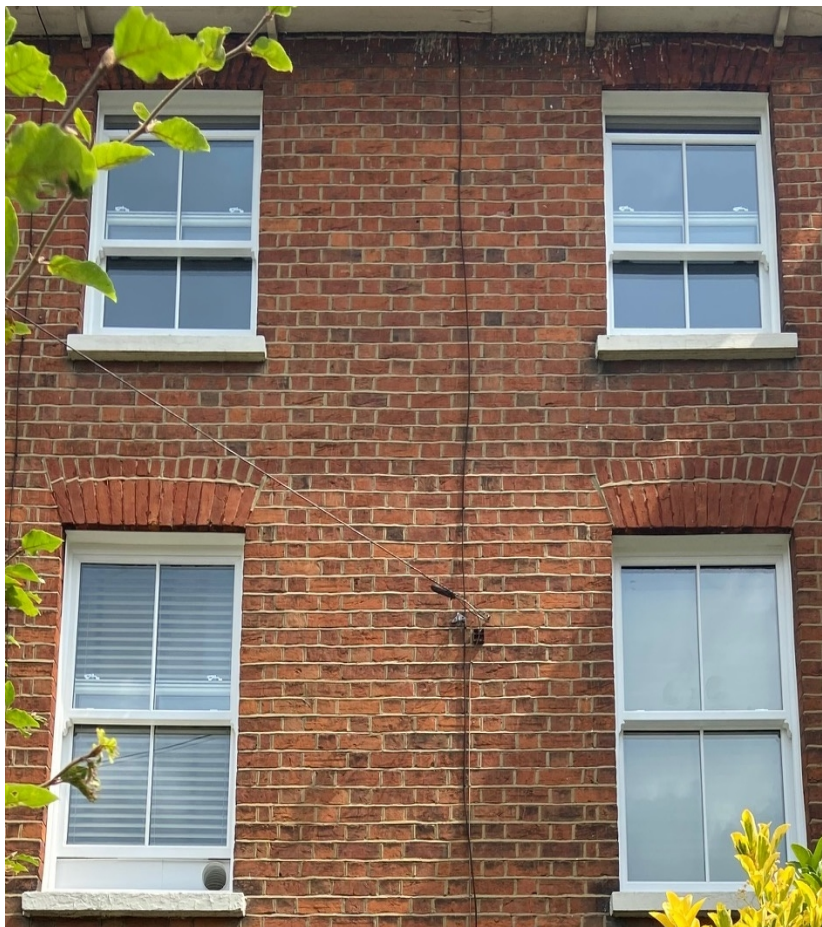
Front of no. 33 with 1 st and 2 nd floor replacement uPVC windows
