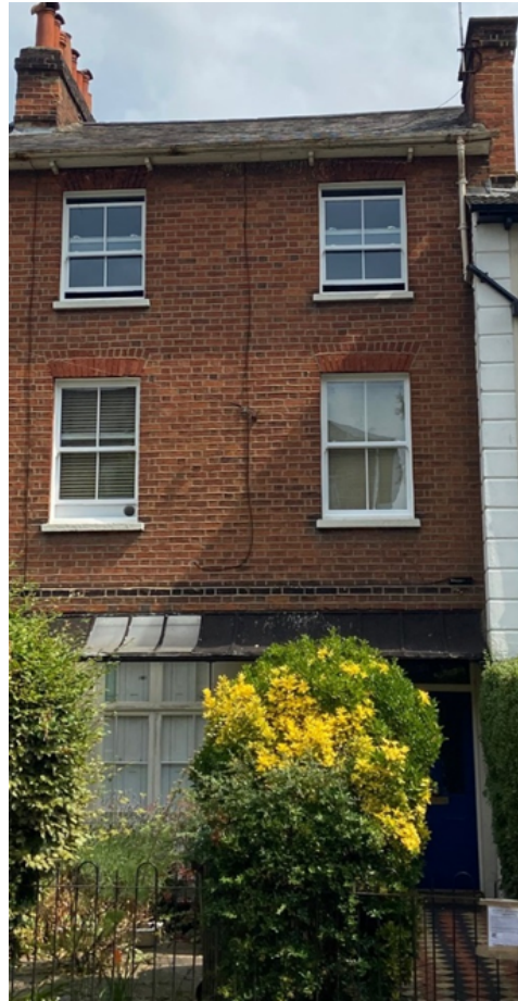
Front of no. 33 with 1 st and 2 nd floor replacement uPVC windows
