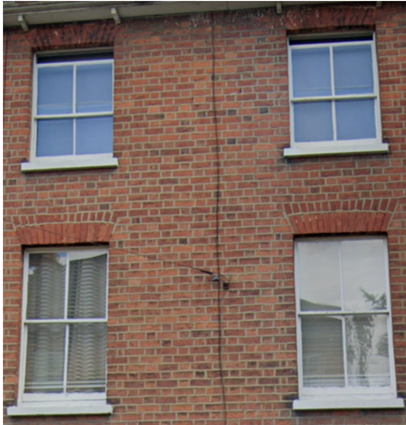
Front of no. 33 with 1 st and 2 nd floor timber windows
