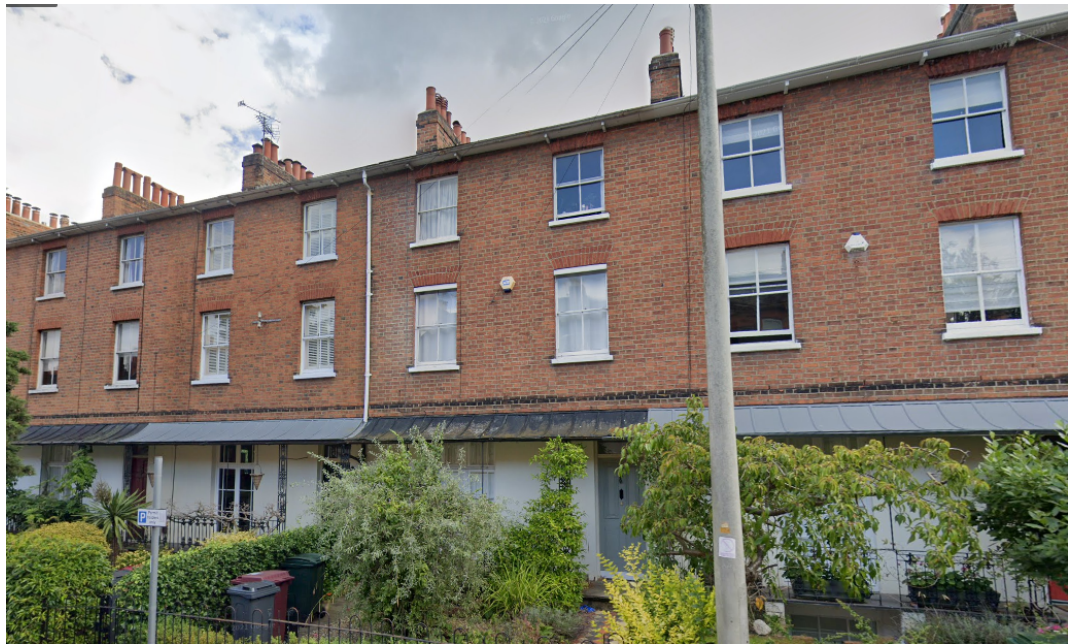
Timber sash windows at no.s 25 to 31 Jesse Terrace
